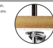
Cut off the excess pipe allowing for a suitable working length to allow for the required 22mm connection. If a push fit connector is to be used then the pipe must be abraded to remove all chrome plating.
